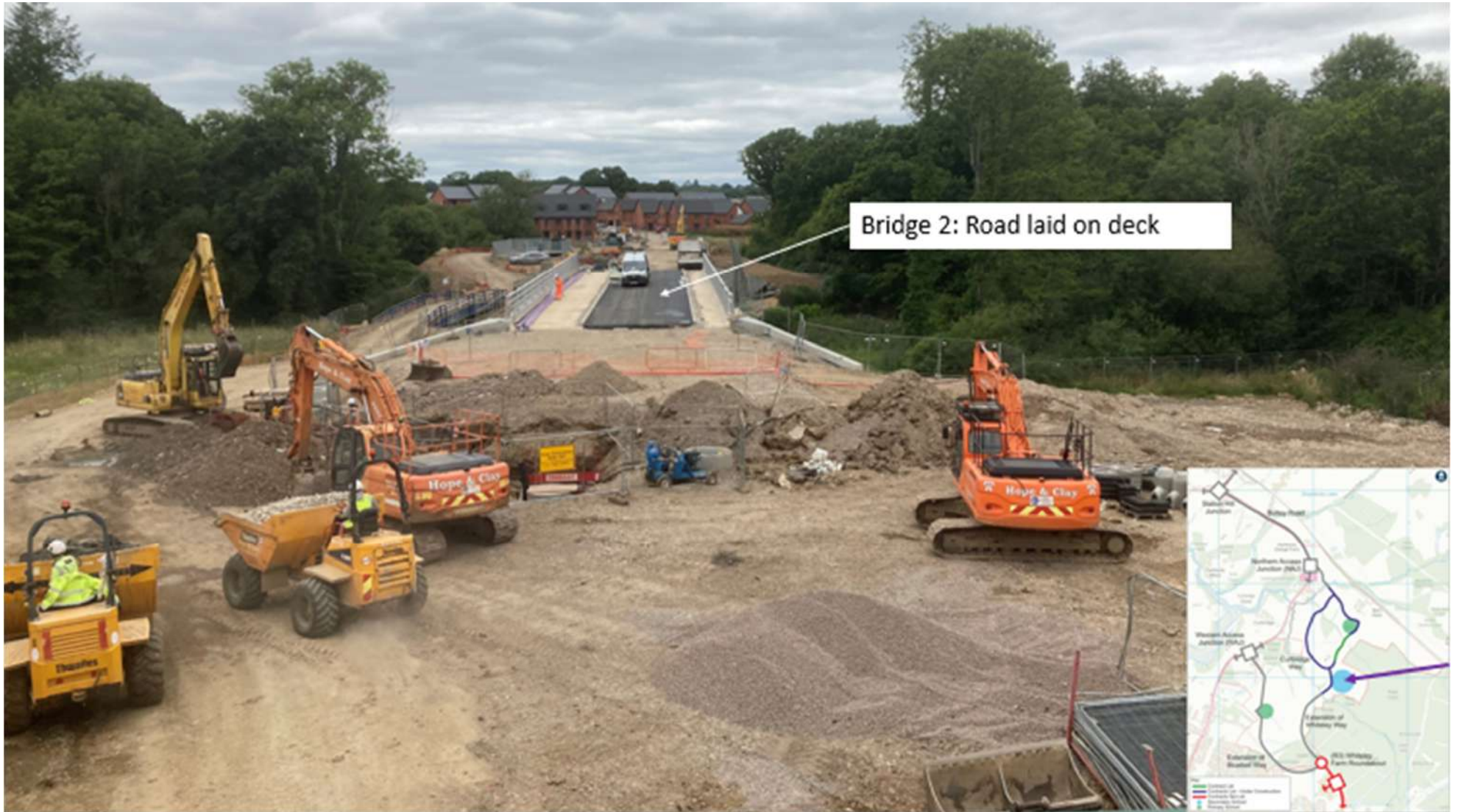
Bridge 2 – Nearing Completion
