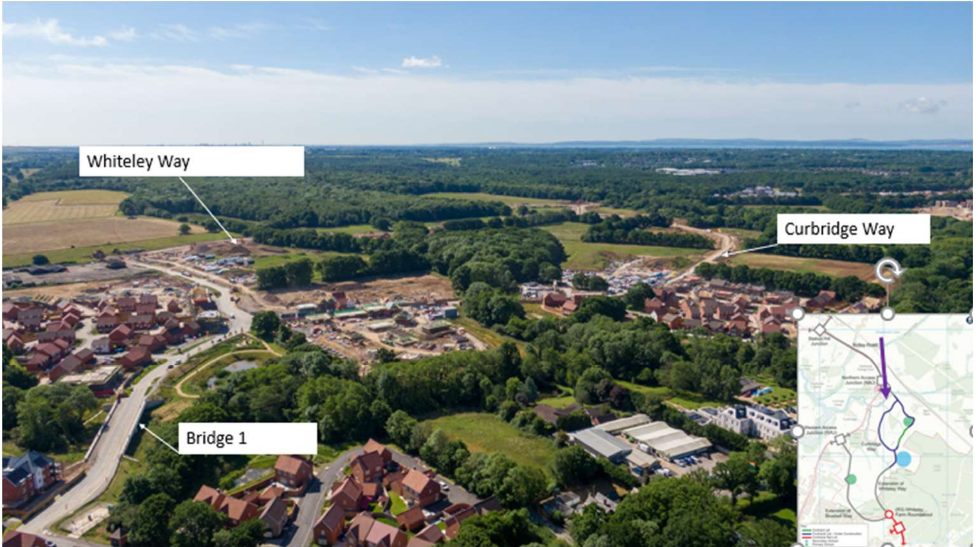
Phase 3 Whiteley & Curbridge Way (View to South)
